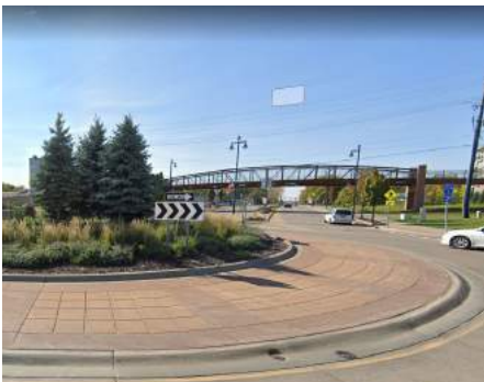
Busy roundabout is an intimidating pedestrian crossing
